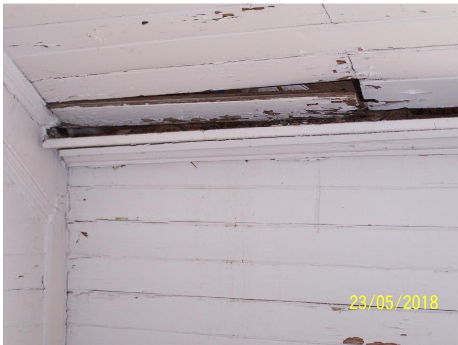
Photograph # 12 – Example of needed wood repairs in the main hall.
