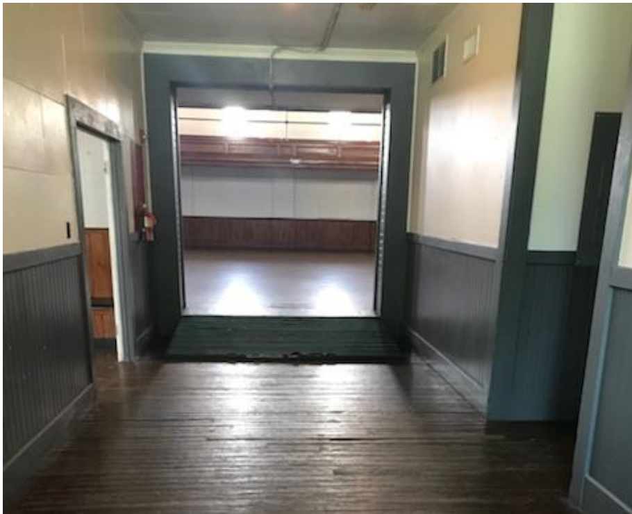
Photograph # 15 – The side corridor showing the ramp leading up to the main hall. The entry door to the Company Room on the left will be relocated to accommodate the new ramp.
