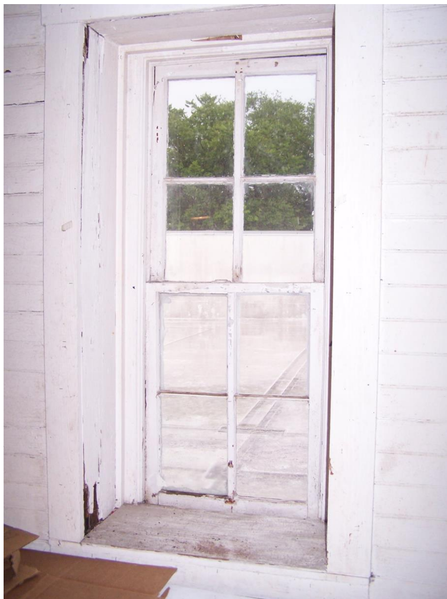
Photograph #16 – Typical window on the upper level of the main hall of Fort Coombs Armory which will be repaired.
