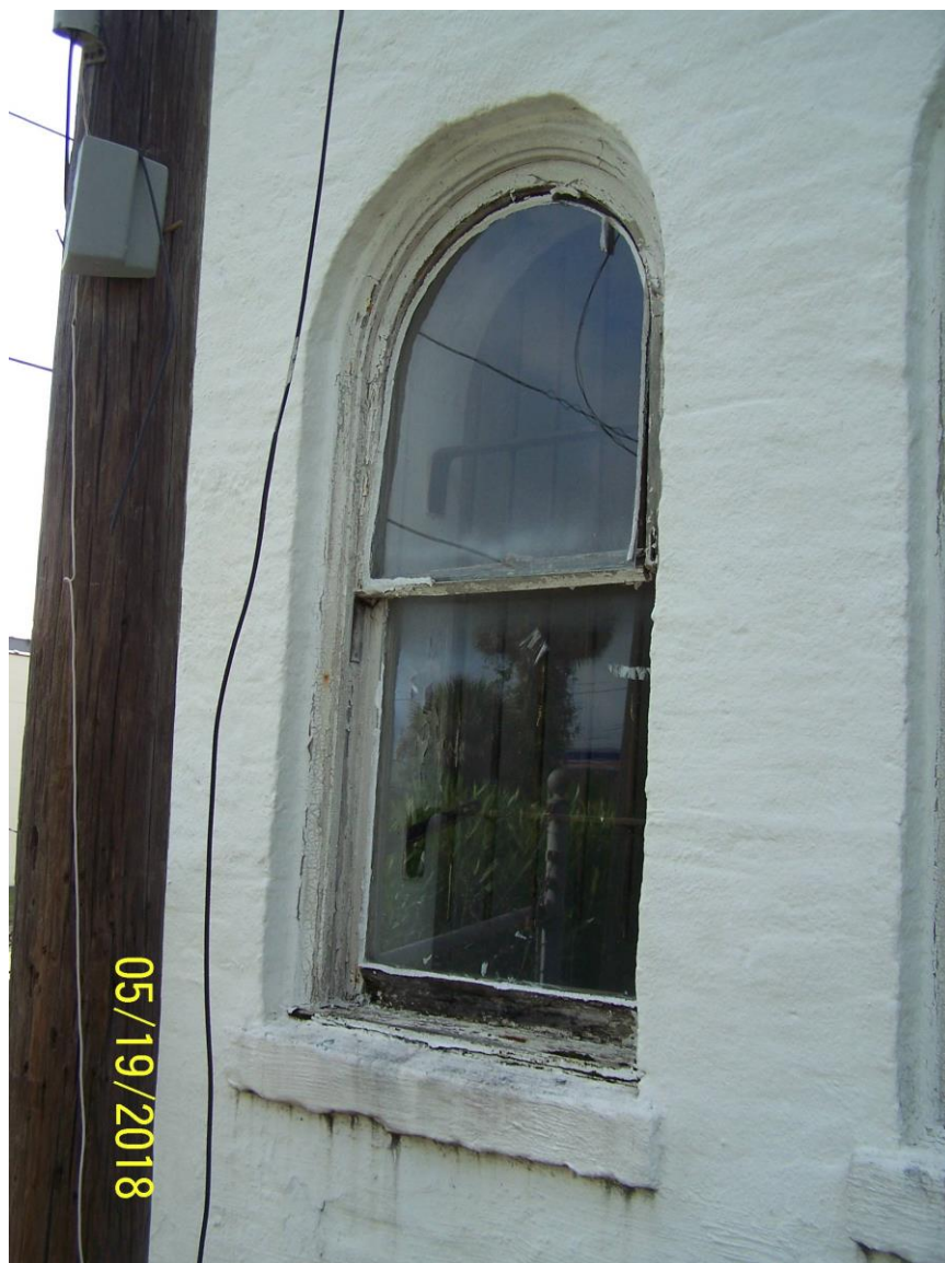
Photograph #17 – Exterior view of a window on the northwest façade of the Fort Coombs Armory that will be repaired. Parts of the sash and frame have rotted away since it was originally built.
