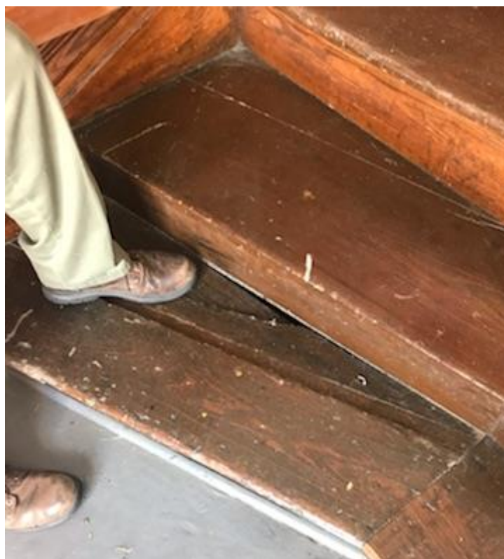
Photograph # 13 – Rotten tread on the stairs inside the Armory that must be repaired.
